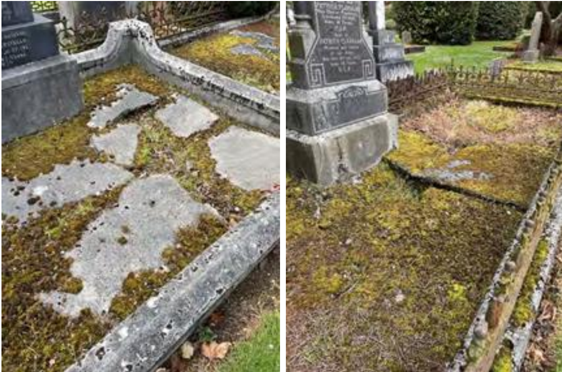
Figure 3 - Grave cut subsidence and memorial on a lean as a result
