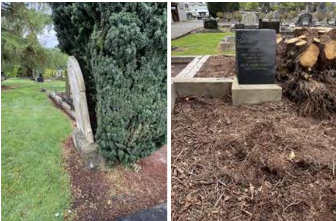
Figure 5 - Vegetation causing memorial to lean/require maintenance
