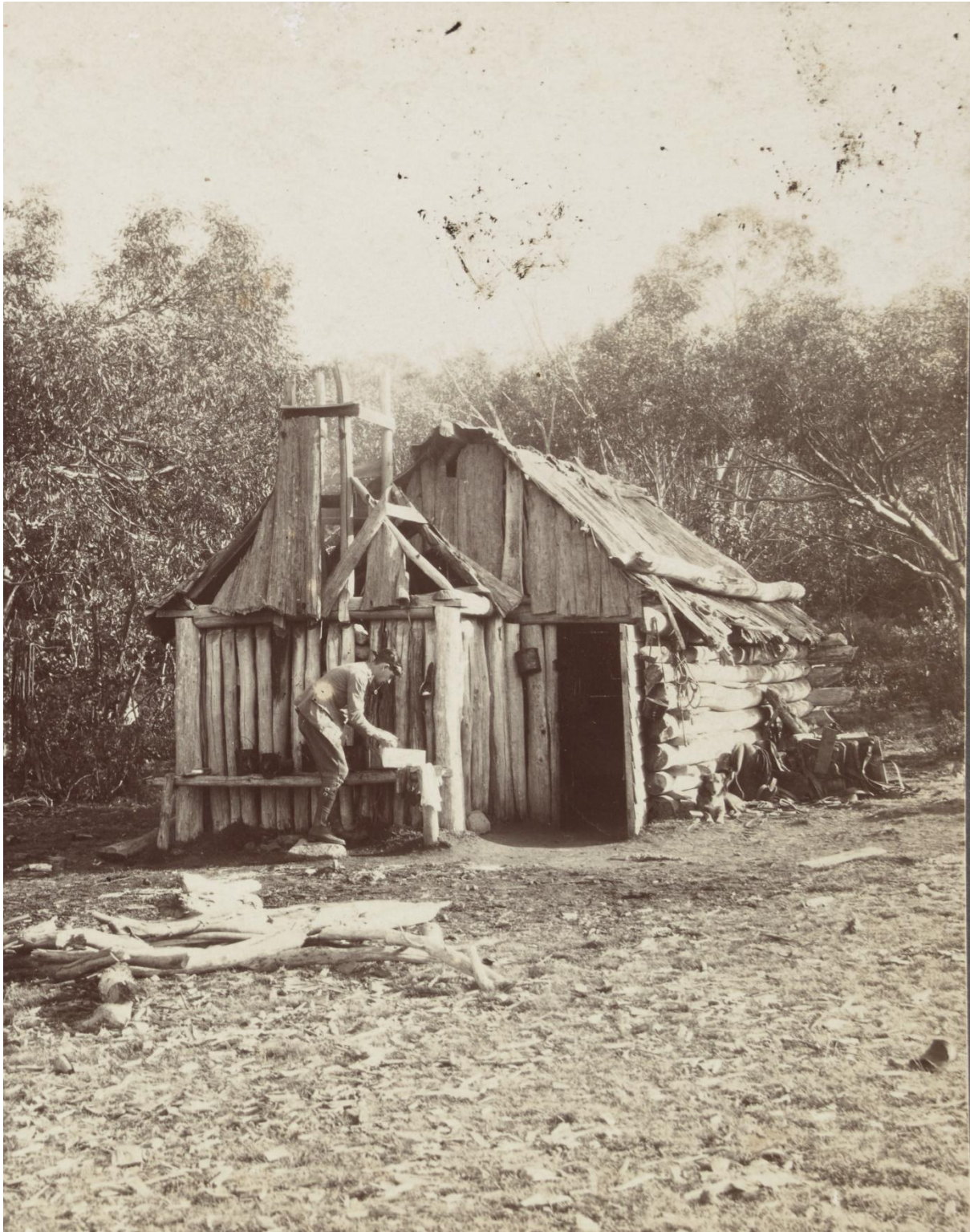
Riggall's Hut near Mt Wellington N. Gippsland, c 1913.
